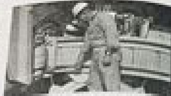
Fig. 22 - Digging the Backhoe into the Right Side of the Trench
