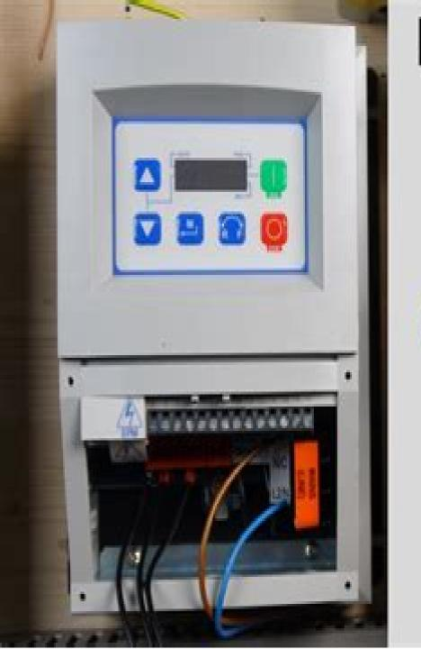
**Lenze SMVector** VFD, **Local control** Commissioning Parameter set up **Factory reset**
