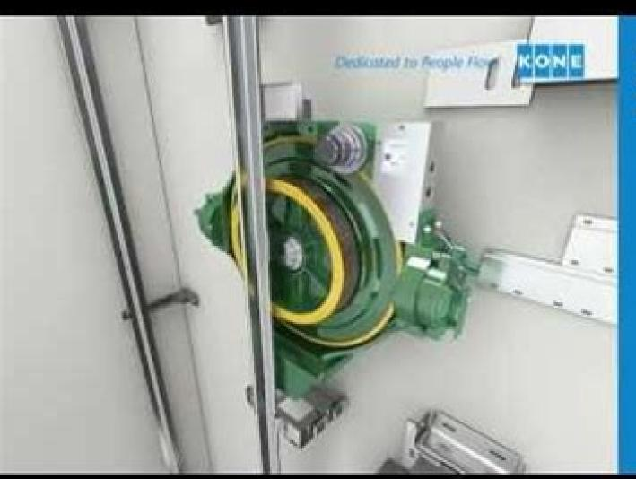
KONE EcoDisc is so thin that it can be placed in the narrow space between the guide rail and the shaft wall
